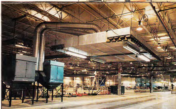
Morris Welding Exhaust System
